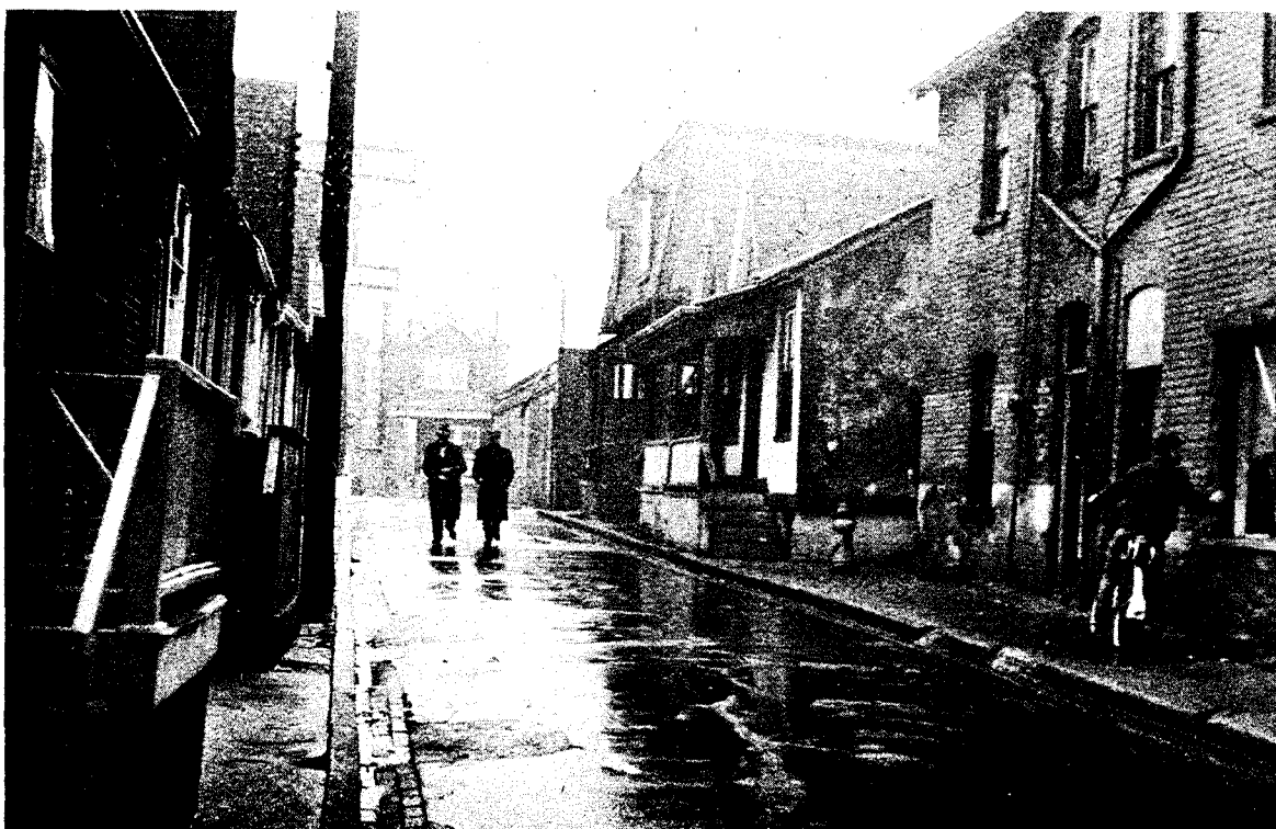
Crumbling streets, traversed only by drunks
